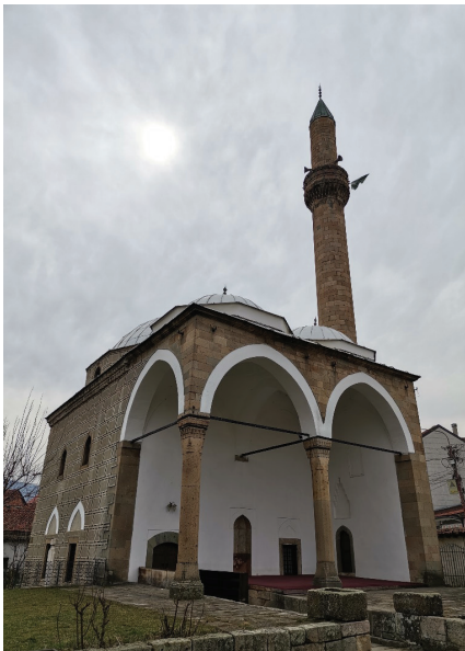
Add. 1. The Altun Alem Mosque before the last renovation, Huseinović 2021.
